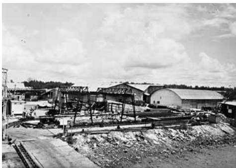
Reconstruction of wharves 4&5, Port Swettenham casting yard for 24" dia piles and 14" x 14" piles 1-12-67.
