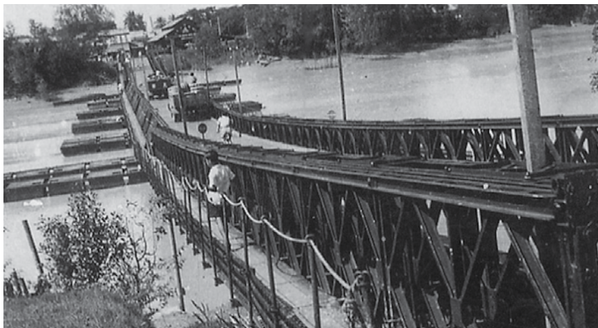
An example of a Bailey bridge. Created by Sir Donald Coleman Bailey OBE during the Second World War, these bridges were meant to be quickly assembled, and were strictly temporary in nature late 1940s.
