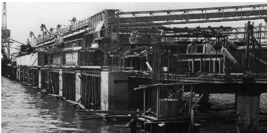
1973 Front face of partially completed wharf joining Wharves 3 and 4.
